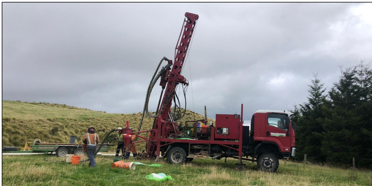
Figure 1 Drilling rig on site at Lammerlaw
